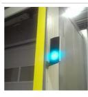
The traffic light system either has a sensor above the dock leveller that measures the presence of the vehicle or it is a wheel chock that detects the vehicle.
