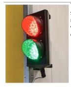
The traffic light system either has a sensor above the dock leveler that measures the presence of the vehicle or it is a wheel chock that detects the vehicle.
